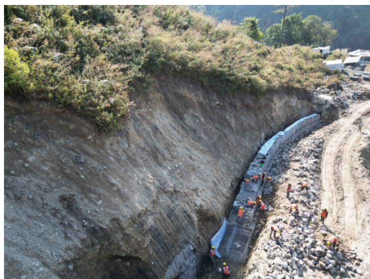
Slope Protection Works at Access Road
